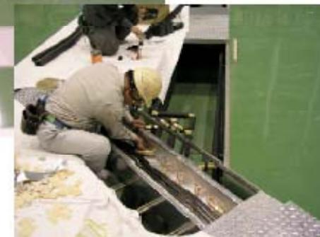
• Insulated duct set in the under-floor cable trench.
